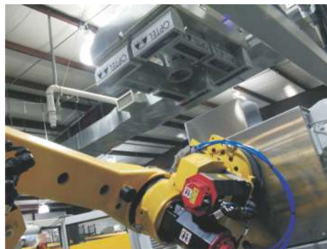
Integrated Overhead Vision System Verifies Case Load
